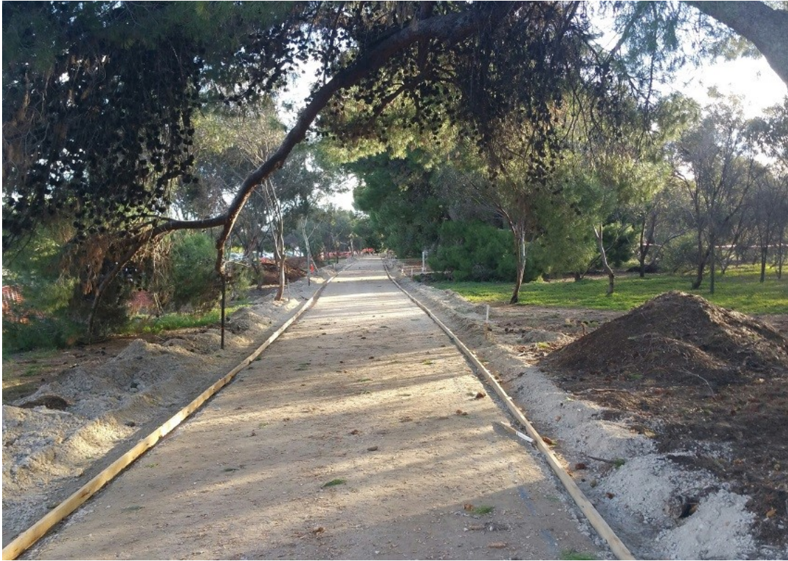
...and currently under construction. (Photo taken on 14 May.)
