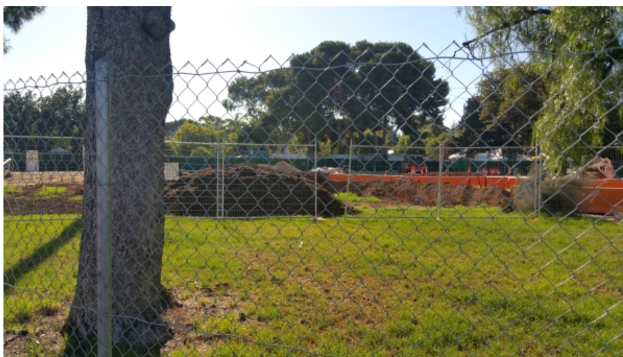
The ongoing sacrifice of Rundle Park (Park 13) to O-Bahn construction
