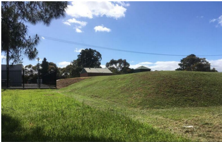
External view from the south-west with the electricity substation in the background
