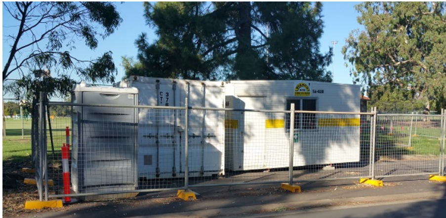
A works compound, taking over part of the University playing fields on Karrawirra (Park 12) off War Memorial Drive
