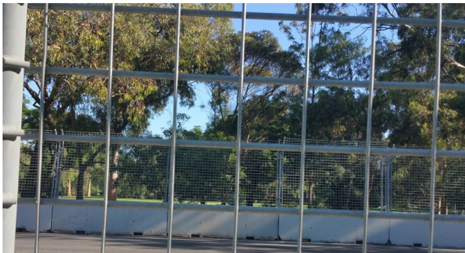
Car racing fences preventing access to Ityamai-Itpina (Park 15) off Bartels Rd
