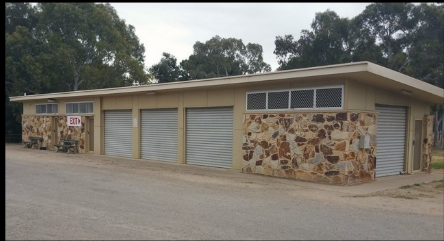
Existing Council horticultural depot
