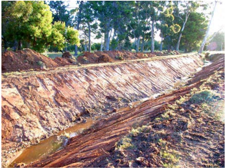
Top and right: Parklands Creek at the southern end of Victoria Park. One week of 'laying back banks' by the ACC resulted in a dangerous and unsightly stormwater drain. Photo taken in April 2006 by Gunta Groves.
