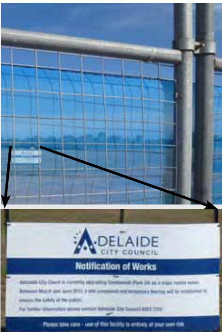
Top: Adelaide City Council notification sign obscured by fencing and blue netting. Park 24 plateau 'Major event' works site west of Adelaide High School / Ellis Park soccer fields carpark from which 2,690 remnant native plants were reported to the Atlas of Living Australia in March 2013. Photos by K Henderson.
