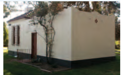
Above: View of the south and east elevations, showing the exterior of the exercise wall yard and holding cell. Source: South Australian Heritage Council Summary of State Heritage Place No 26365, Former Torrens Lake Police Station, Victoria Drive, Adelaide.
